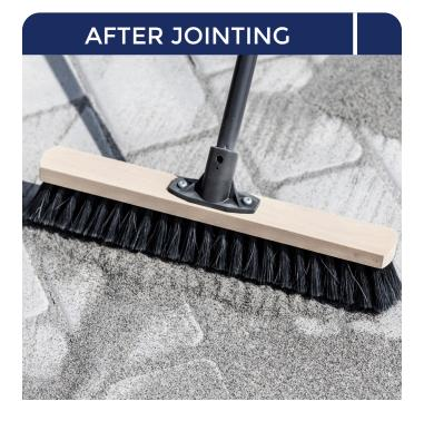
Failure to clean the pavement before watering can result in mortar residue or staining on the surface. Should the unfortunate happen, it can be removed with water and a stiff brush.
