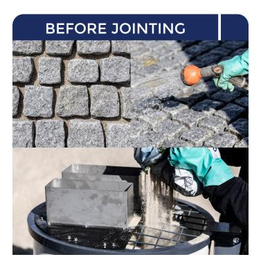
Always start with a small area to see how the pavement responds to the joint.
