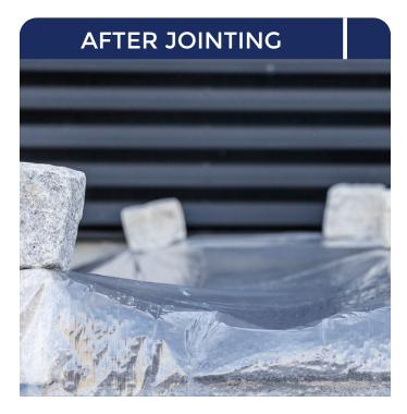
ATTENTION! A thin film will form from the adhesive on the stone surface. This film wears off over time with normal use of the pavement. Strength joint L15 is not recommended for ceramic tiles or sandstone, as the film from the joint is difficult to remove on these surfaces.
