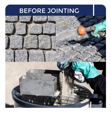
Always start with a small area to see how the pavement responds to the joint.
