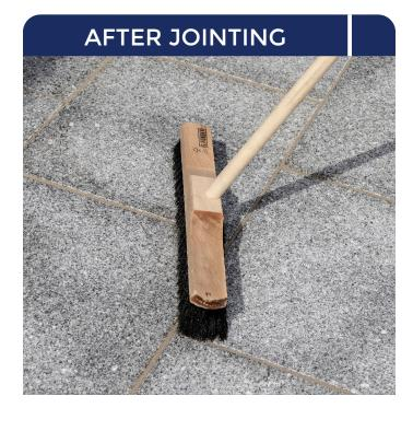
Clean the stones with a soft broom to prevent the jointing material from sticking to the top of the stones.
